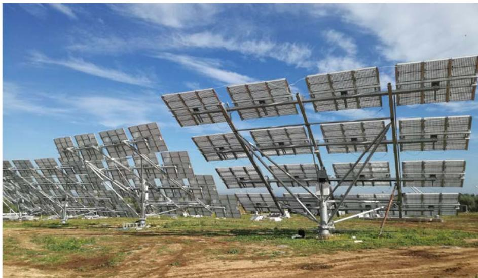
*Applying Solergy COGEM 2-axis Trackers to repower a poorly performing CPV plant*
